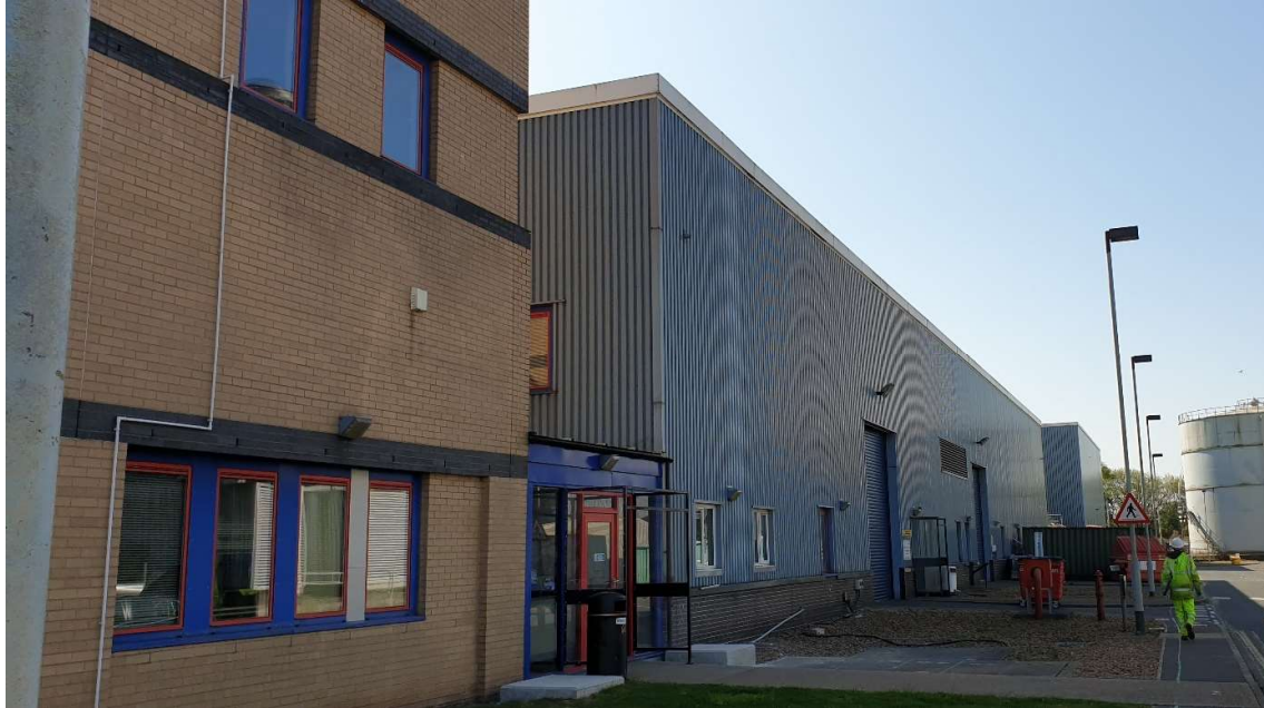
Photograph 1 – The existing Keadby 1 Power Station buildings complex
