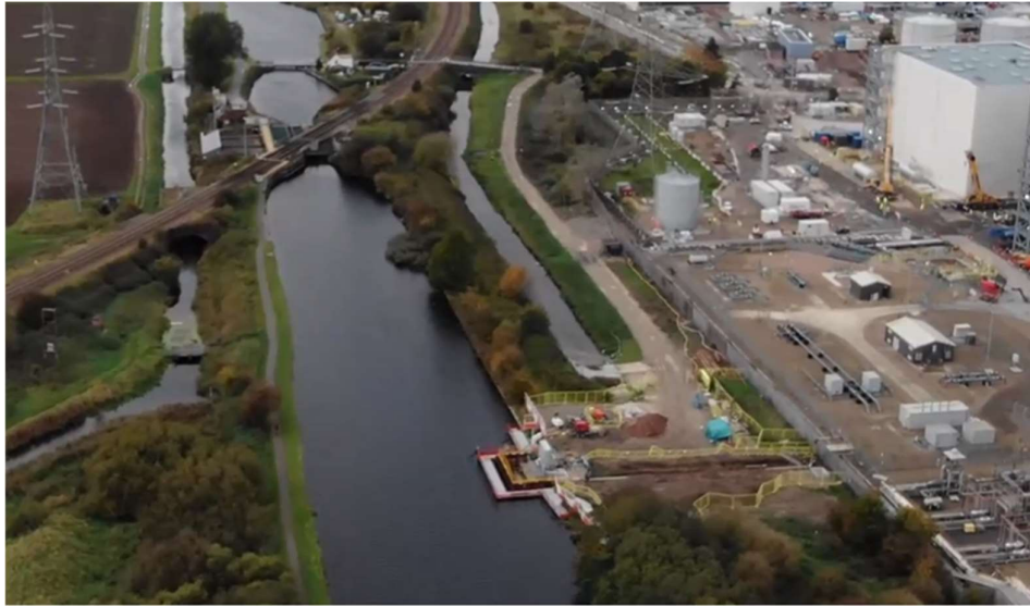
Photograph 23 – Stainforth and Keadby Canal looking over the construction site for the Keadby 2 Power Station water intake (November 2020)
